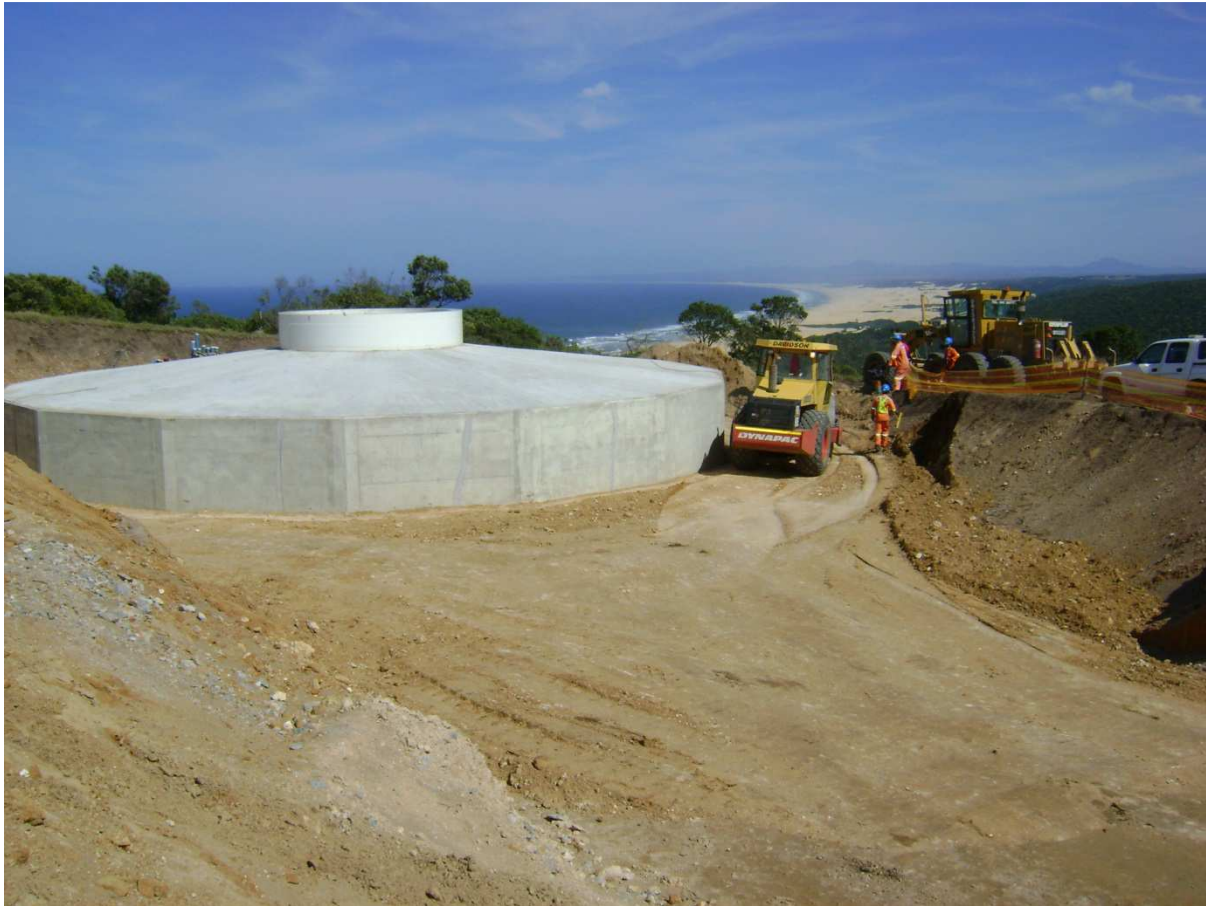
Turbine concrete foundation being backfilled and compacted
