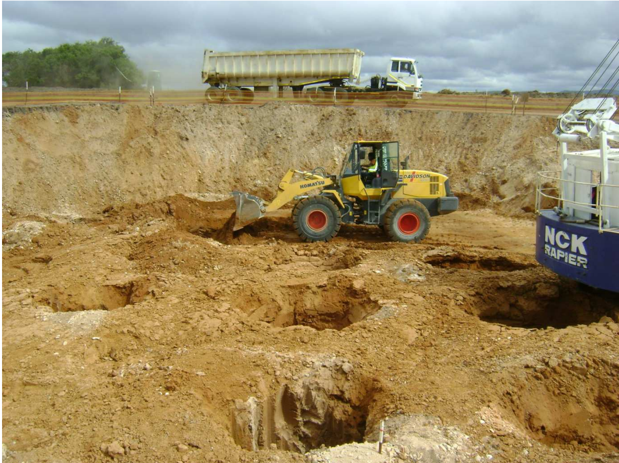
Turbine base excavation showing dynamic compaction imprints prior to being backfilled
