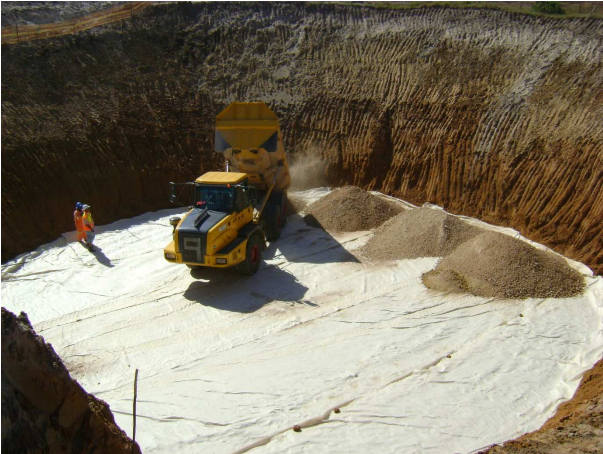
Turbine foundations after placement of Triaxial Geogrid and commencement of engineered layer-works
